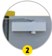
2 Self-closing door with thermo-fuse
