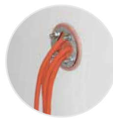
Drilling for cable passage PEXTBALI
